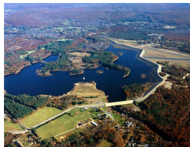
Mansfield Hollow Dam (Credit: ACOE)
