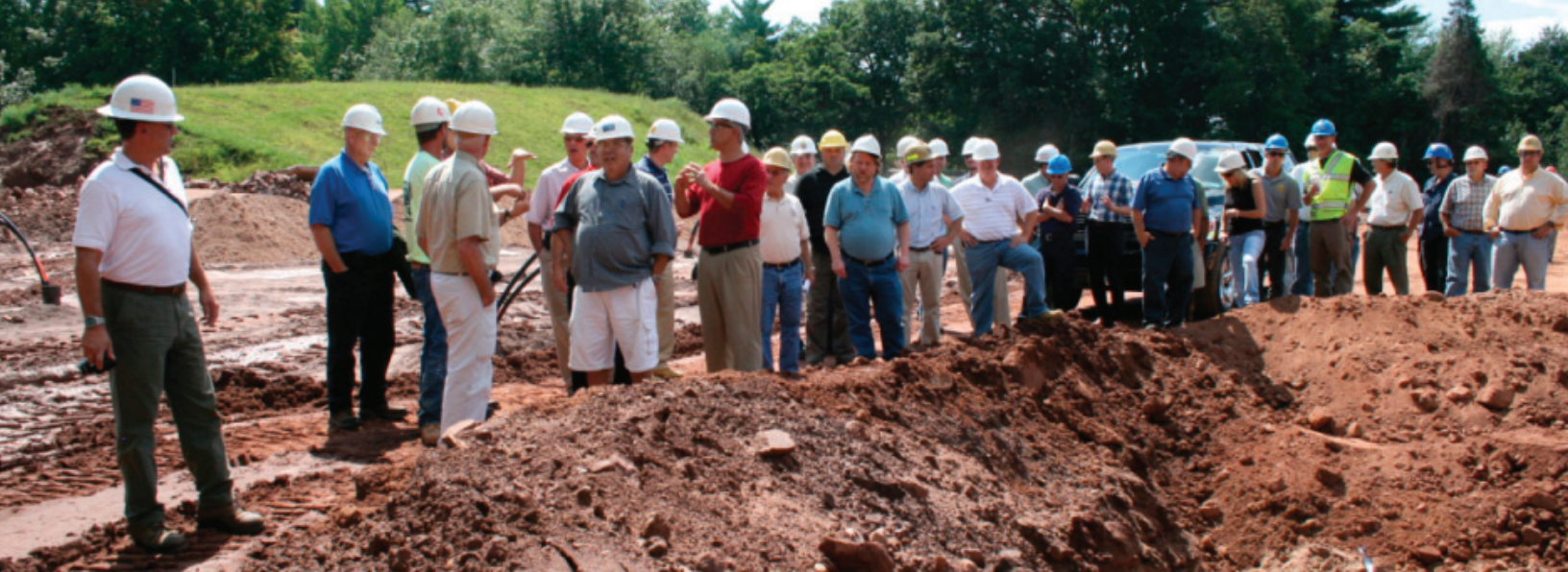
Geothermal instructor Peter Governale leads a site visit of the well field at Forestville Elementary School in Bristol, CT, during ISE's code training on renewable energy systems for local building officials. Funding provided by the American Recovery and Reinvestment Act.
